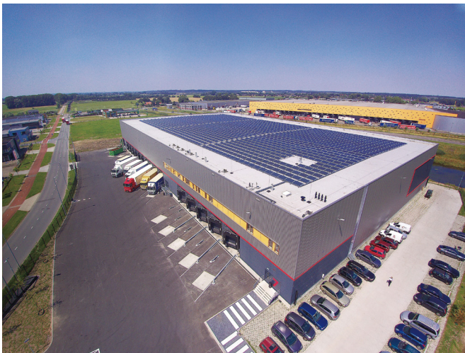
Onsite solar installation at the Retail division's logistics centre in Heteren, Netherlands
