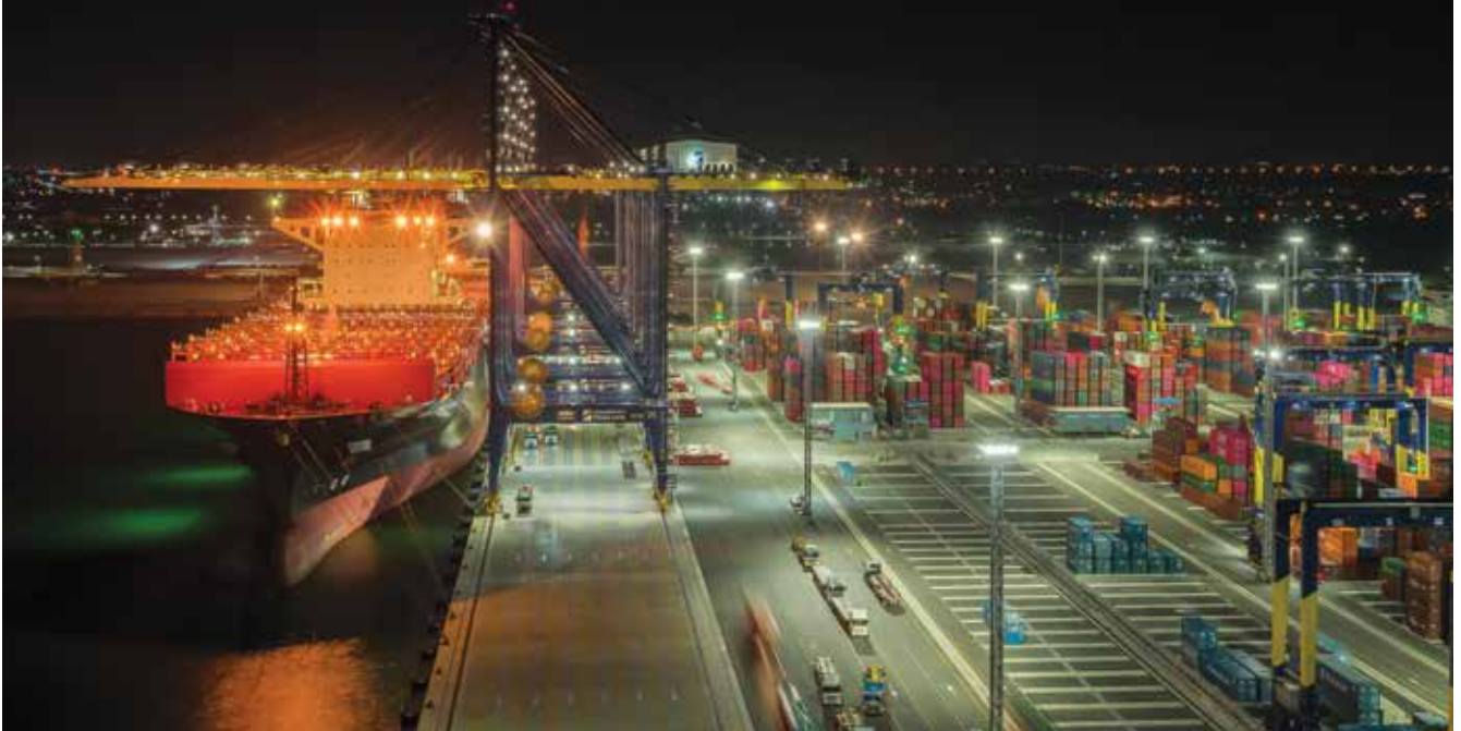
Lighting and camera technology deployed by Hutchison Ports Thailand creates a night-time working environment that allows for maximum performance around the clock.
