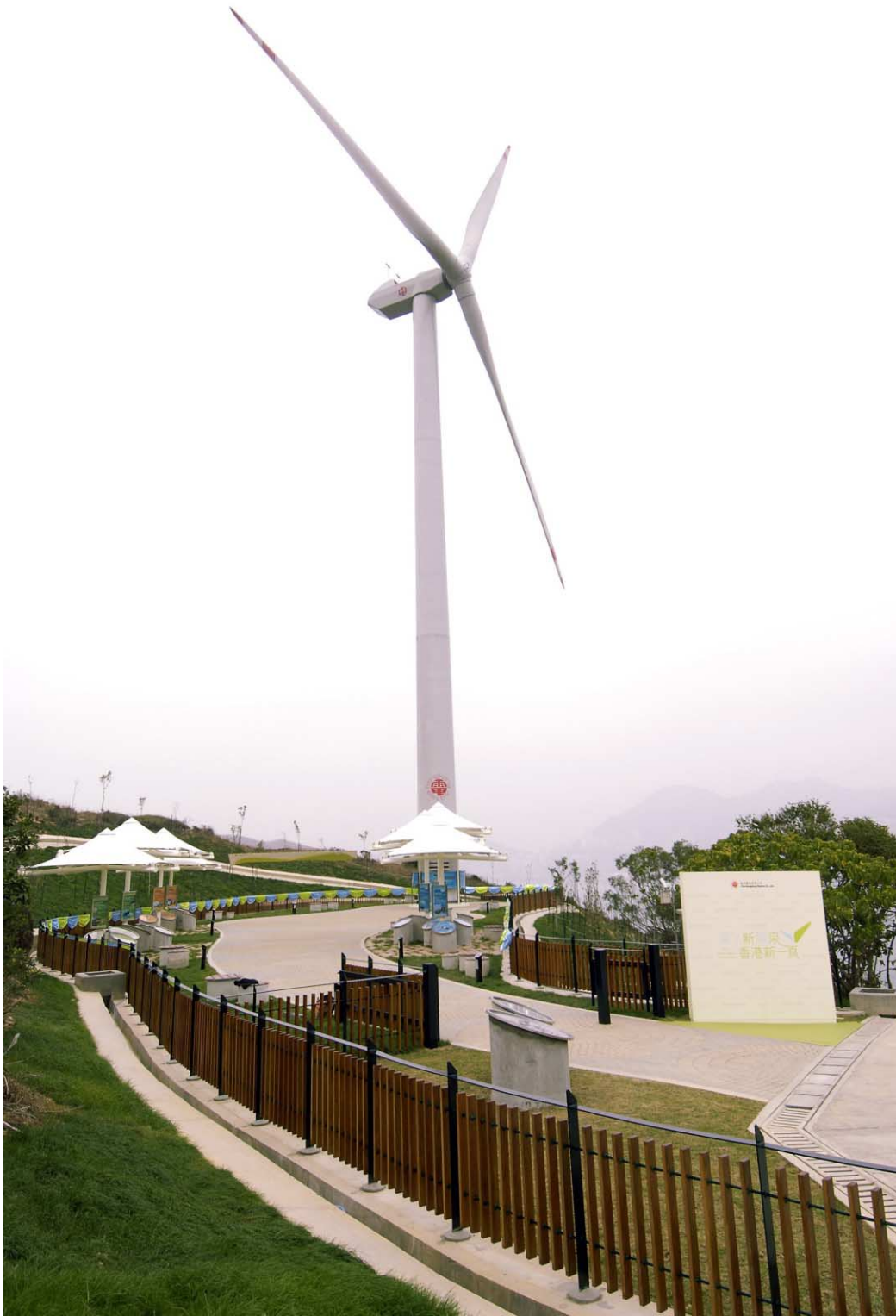
5. Lamma Winds , the first commercial-scale wind power station in Hong Kong.
